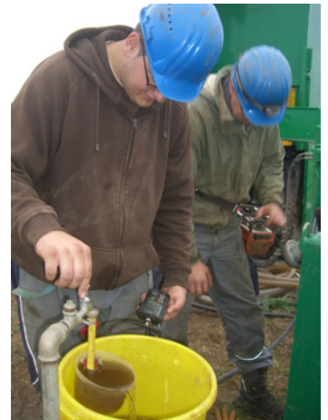
Figure 2: Process control of hydraulic-chemical rehabilitation. © Rudolf Lange Brunnenbau KG, 2013
