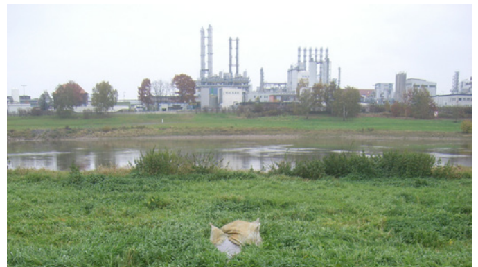
Figure 4: Discharge out of the well. © Rudolf Lange Brunnenbau, KG 2013
