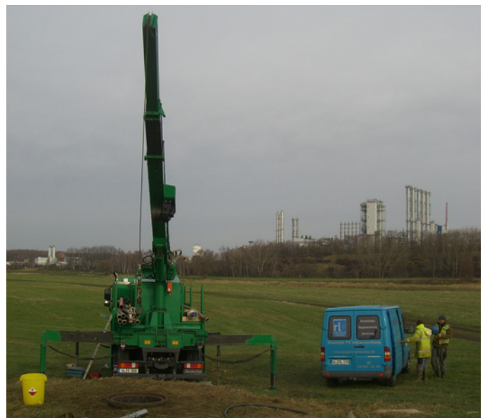
Figure 1: Well site on the river bank. © Rudolf Lange Brunnenbau KG, 2013
